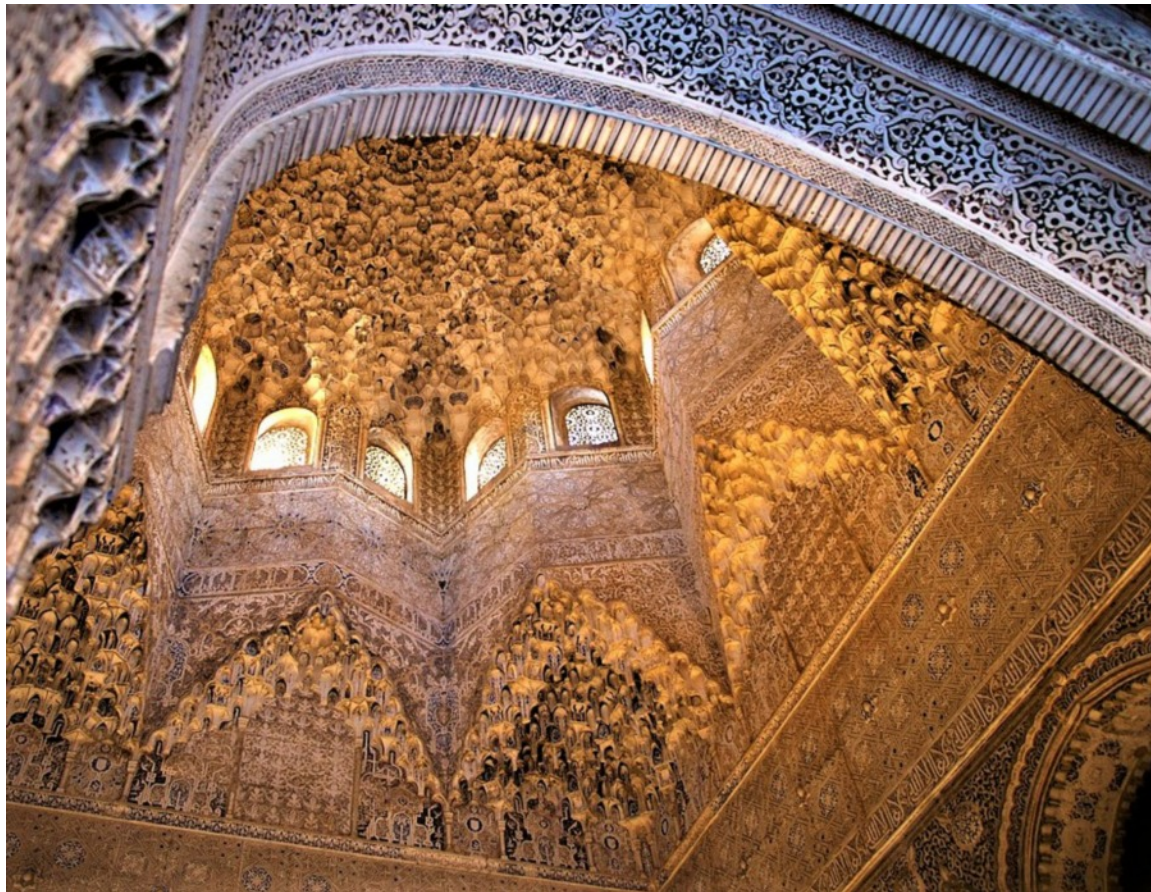
Moqárabe or "stalactite vaulting," Hall of the Abencerrajes, Alhambra Palace – Author, Vaughan Williams, Wikimedia
