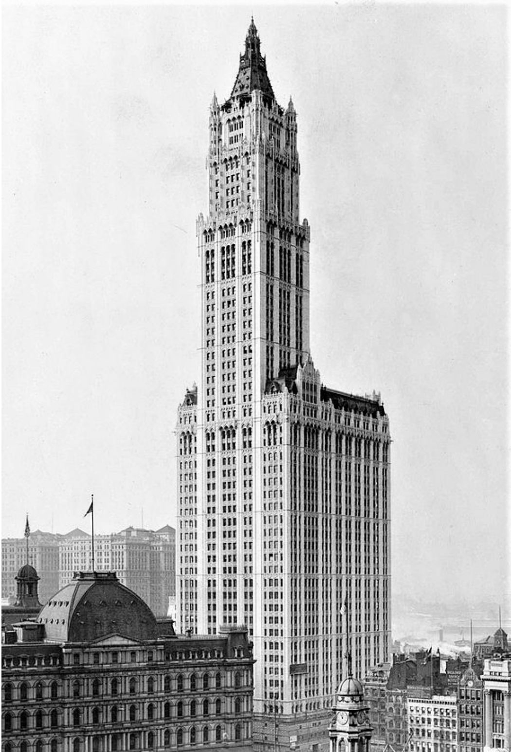
Woolworth Building, New York City, 1913 – Author, The Pictorial News Co., Public domain, U.S. Library of Congress. Designed by architect Cass Gilbert, the 792 foot high 60 story Woolworth building was the tallest building in the world from 1913 to 1930 and remains one of the 100 tallest buildings in the United States.
