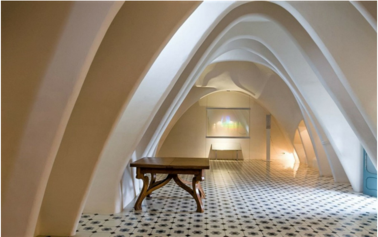
Catenary arches in the attic of Casa Batlló – Author, Sara Terrones, Wikimedia
